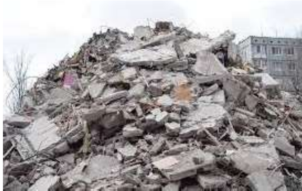
Fig. 6. Construction Site Waste
